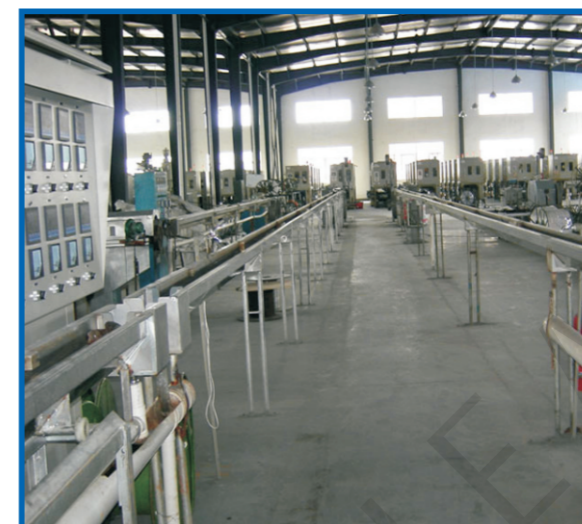
Core Injection Line
